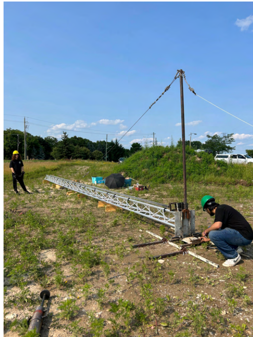
Figure 133: Assembled Launch Tower
