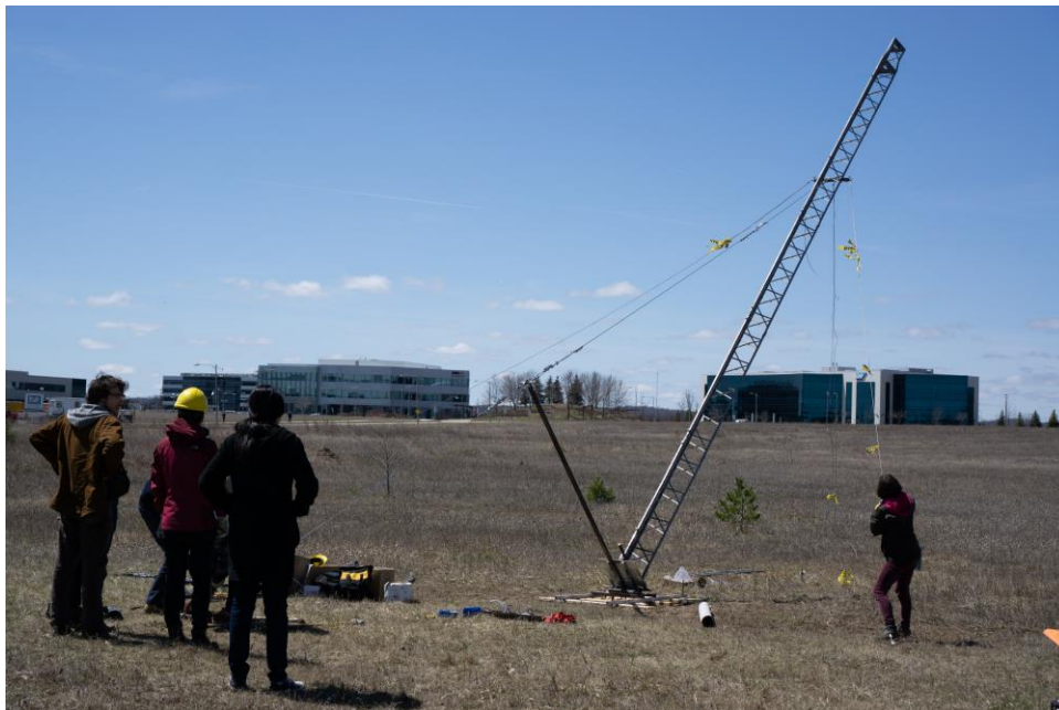
Figure 14. Raising the launch tower to a vertical position.
